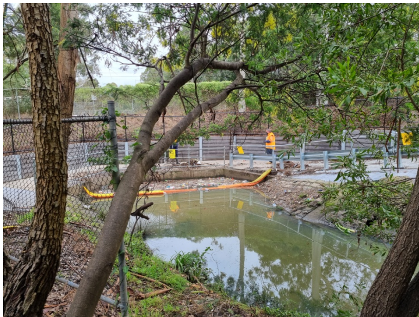
Workers clearing boom of litter, upstream side
